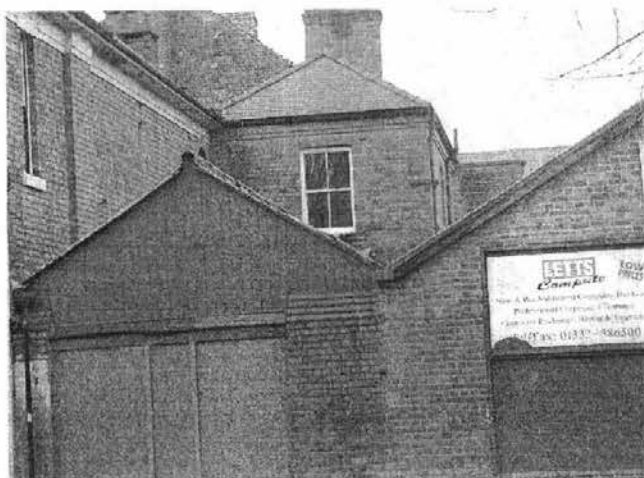
Mr Grundy's 1891 over-roofing to left and Batterby & Hefford's 1942 over-roofing on right Note kitchen extension built by Mr Grundy in 1886. Viewed from King Street 2002.
