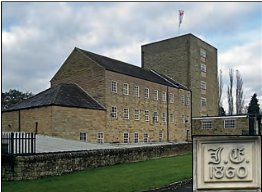
Warney Mill today, as incorporated into the DFS complex at Darley Dale; inset: date stone from 1860 marking the building date and bearing John Else's cypher. [Judith Cooper]
