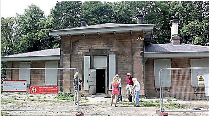
Wingfield Station with its new roof.
