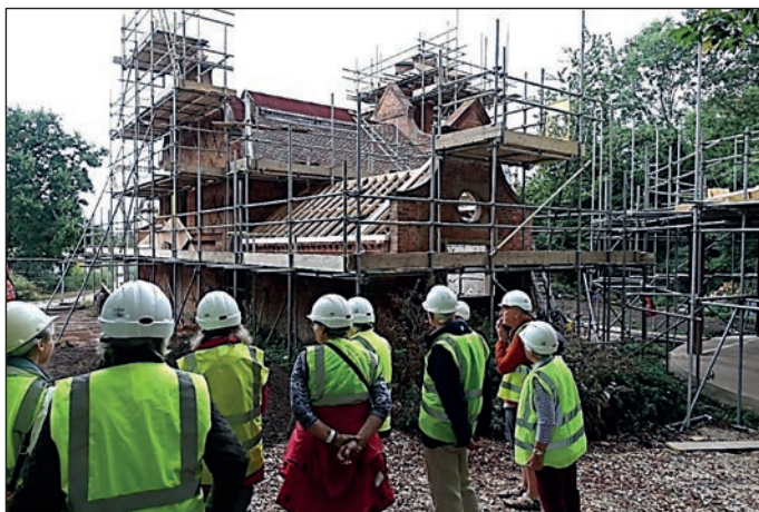
Restoration of the retort house at Sudbury gasworks.
