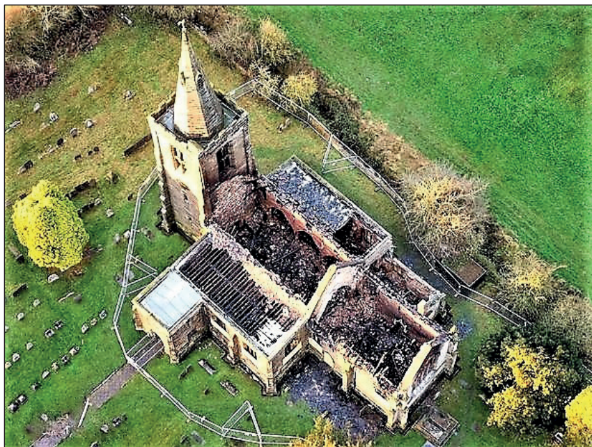
Mackworth, All Saints' church from above, looking NW
