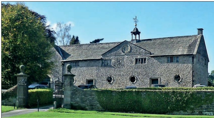
Tissington Hall, stable block, east front, 9 th September 2015, showing the clock dial and wind vane. [M. Craven]
