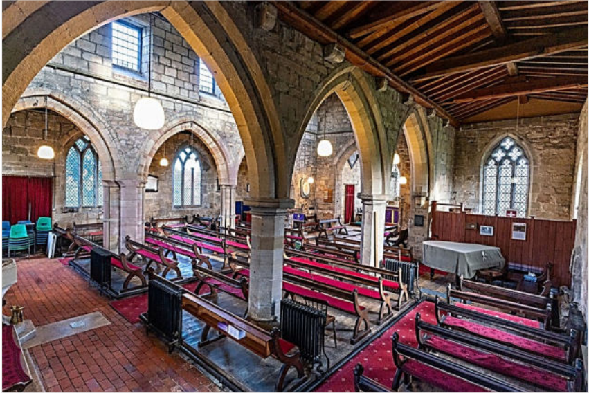
Above: the interior of St Wilfrid's from the south-west before work began: a legacy of 19 th century change and heating systems.
