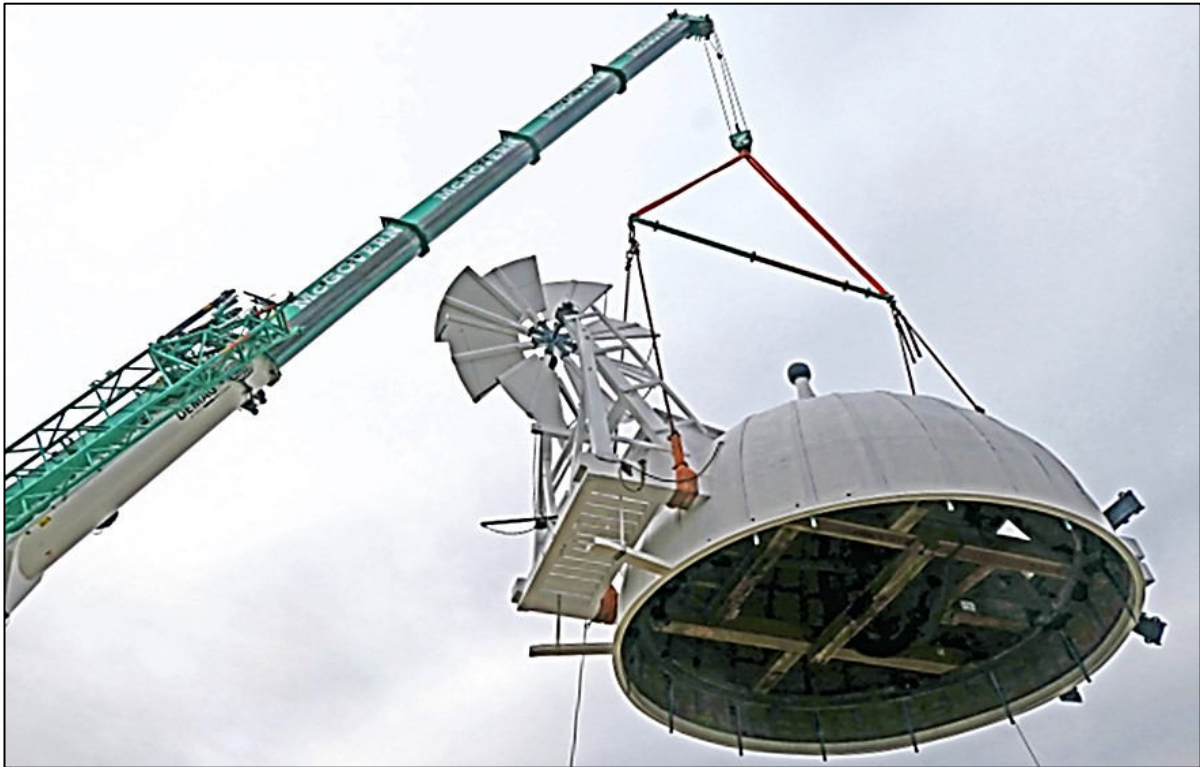
Caps off! – removal of the rotating cap of the mill
