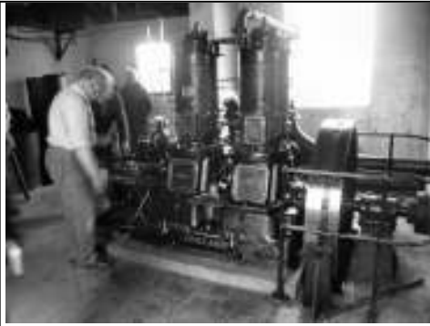
Starting the pumping engine
