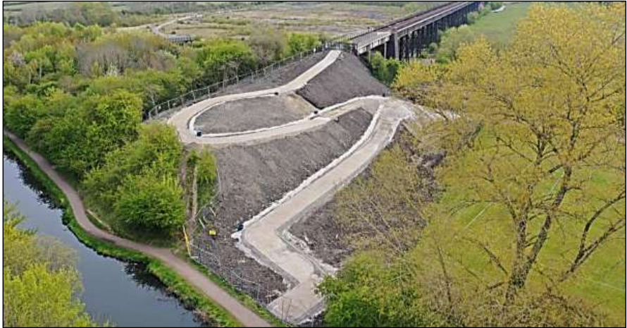
The new western ramp linking the viaduct to the Erewash Canal towpath
