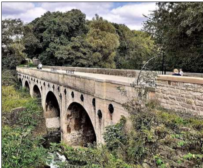
Mansfield and Pinxton Railway: King's Mill viaduct looking towards Mansfield. [Wikipedia]
