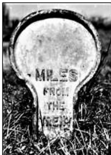
Cast iron mile-marker, Little Chester, photographed by the late Roy Hughes, c. 1960. [M. Craven]
