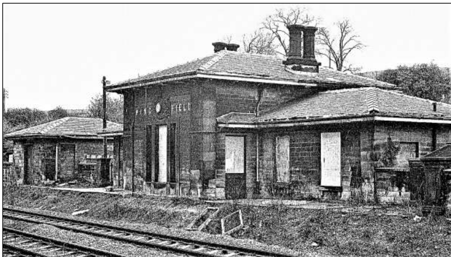
Wingfield station seen derelict c. 1970, when still in reasonably sound condition. [MR Trust]
