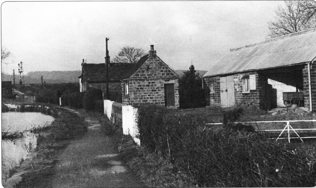
Cromford Canal at Codnor Park c.1955
