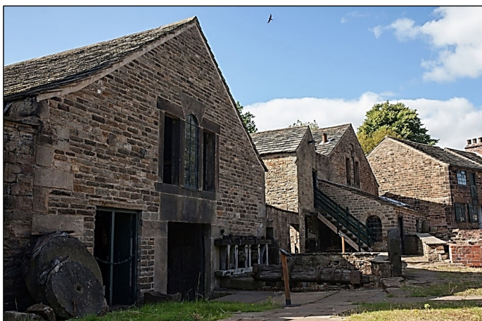
Part of the site, 2021.
