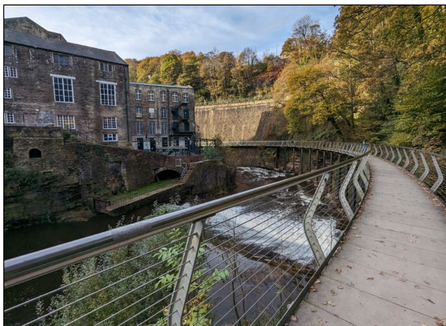
New Mills, part of the Millennium Walkway, 2024.
