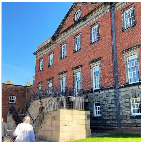
Radbourne Hall, the new stone perron, not quite touching the north front of the house: 2024.
