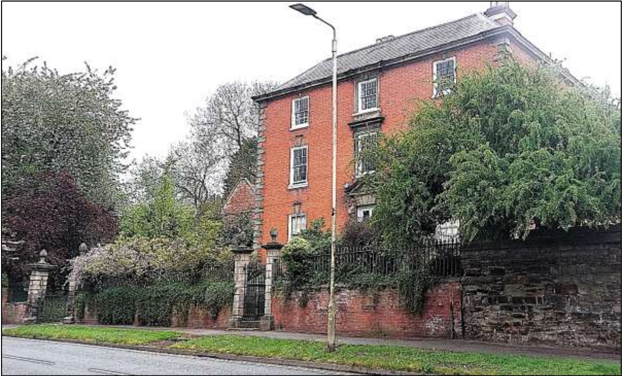
Above: Dalby House, 70-72, High Street
