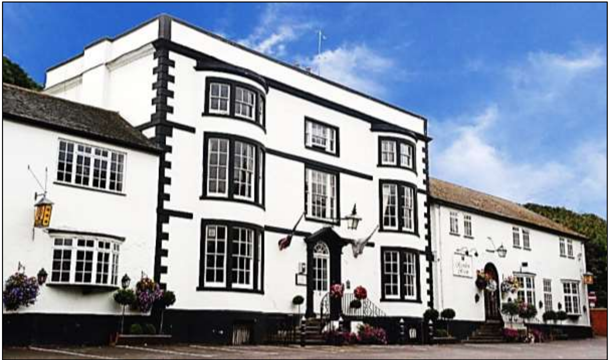
Castle Donington, Manor House, street façade.
