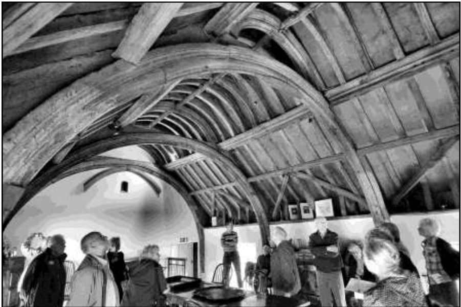
The roof of Cadhay House
