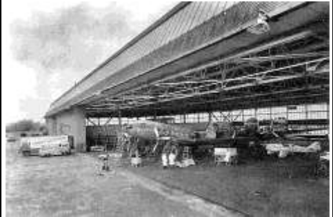
The Derby Airways Hanger at Burnaston Airport
