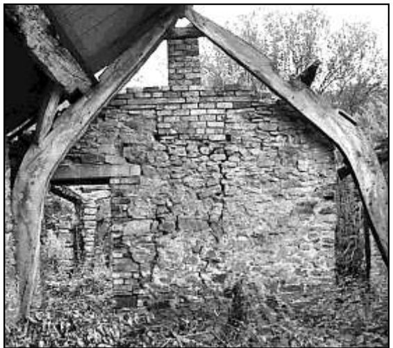
An unloved Cruck Frame in New Mills. 2005
